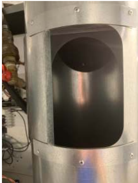
FIGURE 3- Dryer Exhausting Using A Main Discharge Duct
