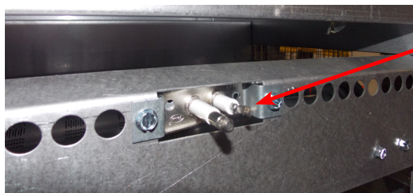
Spark Electrode Located Right side of Burner
