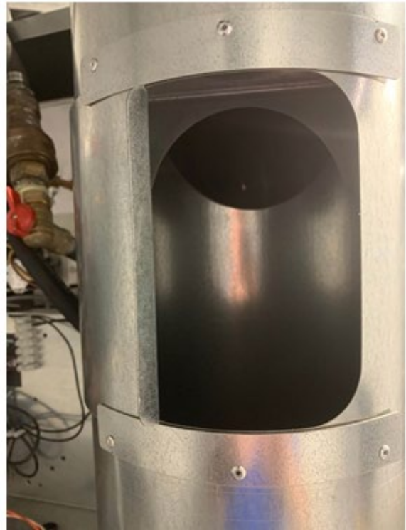
Slide open for routine cleaning
